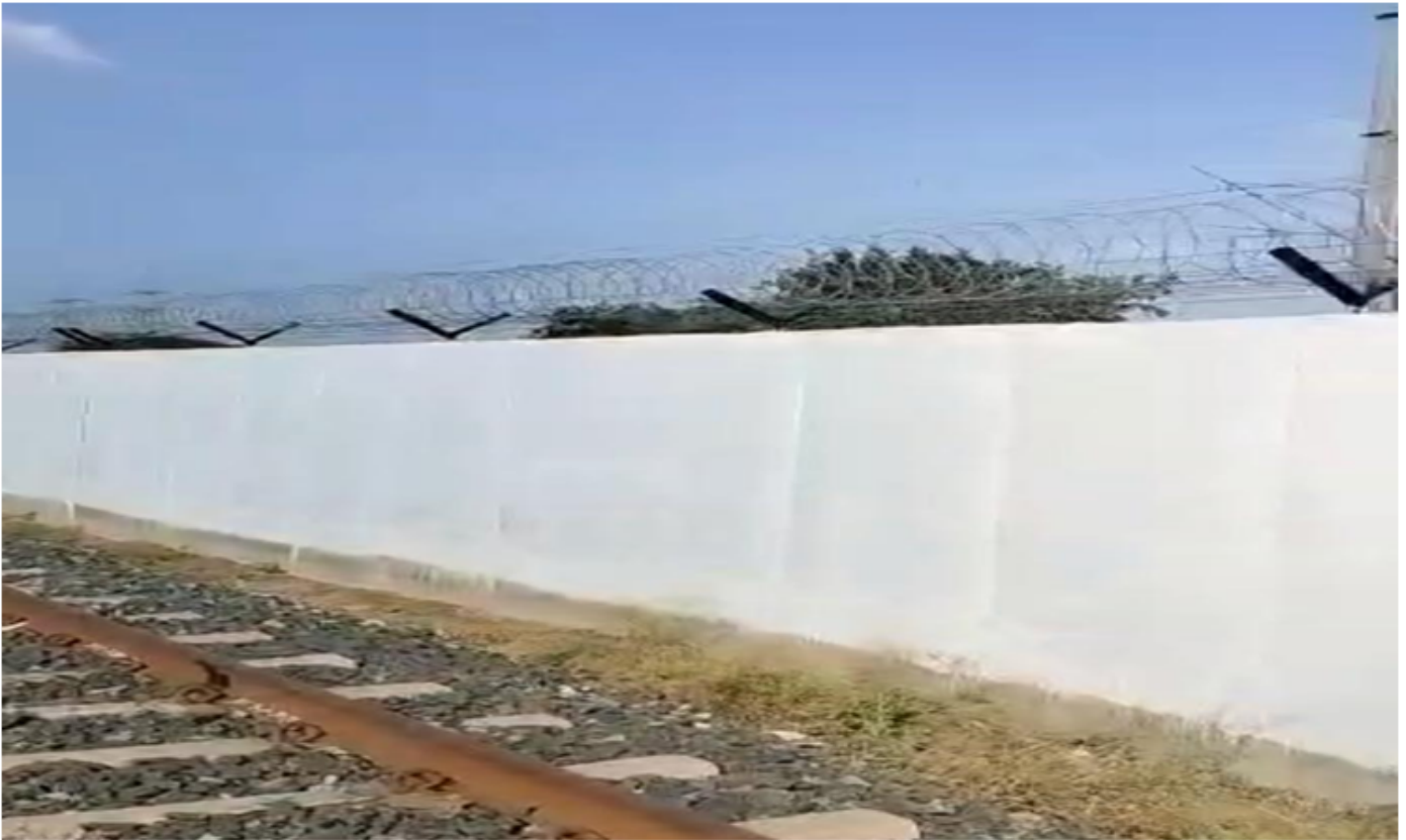
Site Location Of Railway Coach, Badnera (16 zone system)
